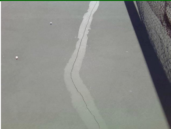
Tennis Courts: cracks & repairs
