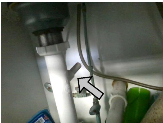
Office/Kitchenette: leak in drain
