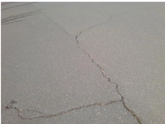
Parking Lot / Driveways: typical cracking
