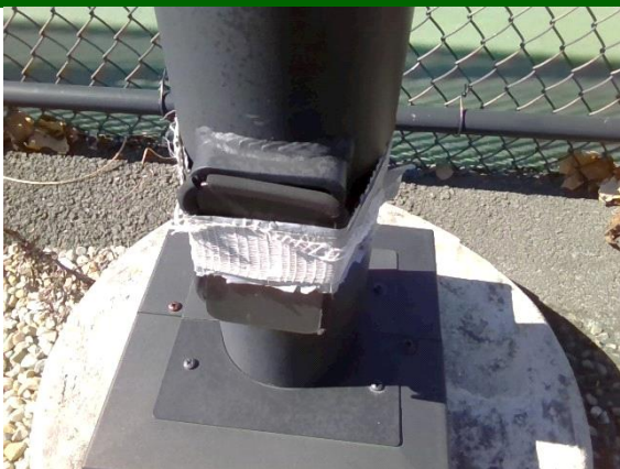
Exterior Surface: damaged standard
