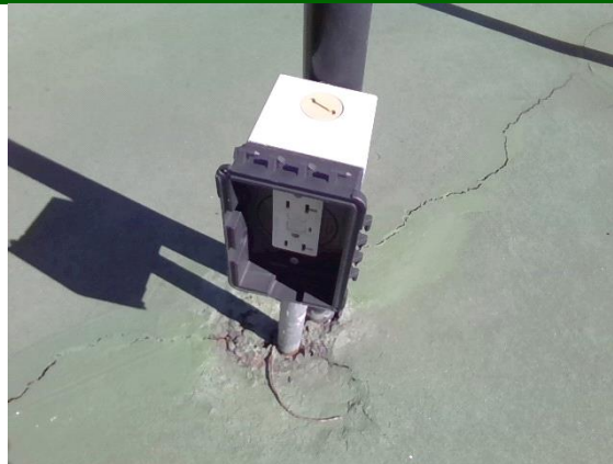
Tennis Courts: damaged GFCI outlet
