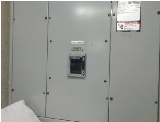
Electrical: service disconnect
