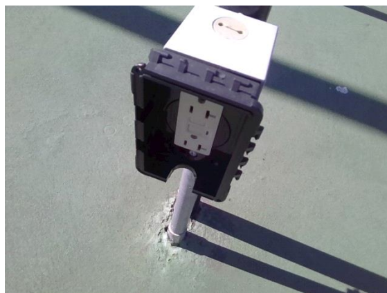
Tennis Courts: damaged GFCI outlet
