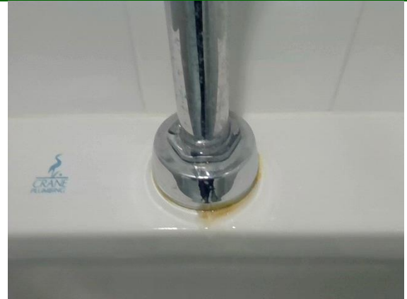
Mens Locker Room: leaking flush valve
