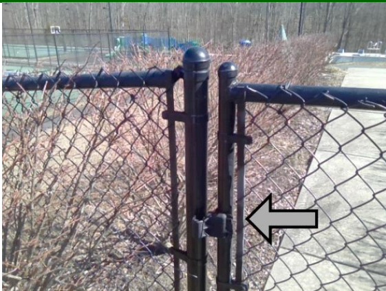
Fences / Enclosures: damaged gate latch
