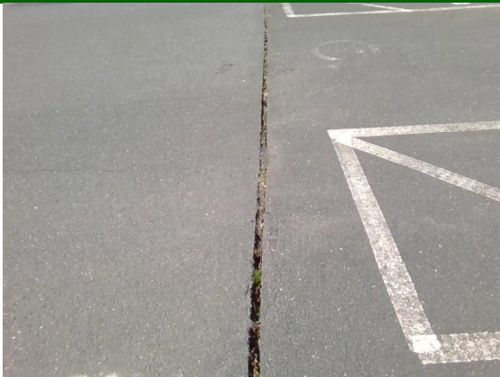
Parking Lot / Driveways: cracked seam
