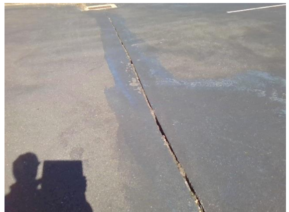
Parking Lot / Driveways: cracked seam
