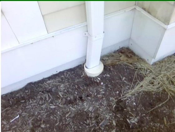
Roof Drainage System: connection below grade
