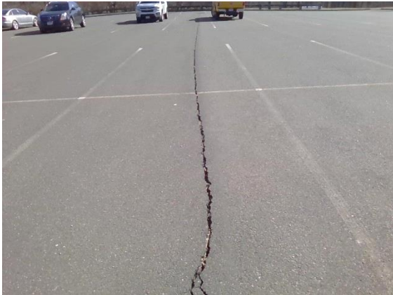
Parking Lot / Driveways: cracked seam
