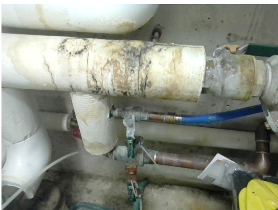
Plumbing: evidence of leaking
