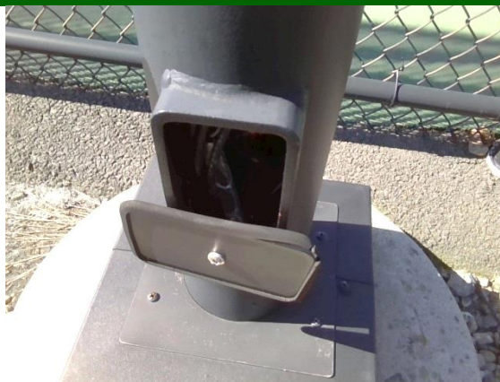
Exterior Surface: damaged standard
