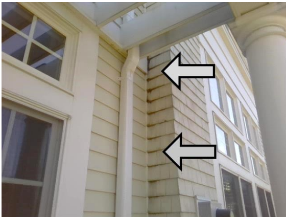
Roof Drainage System: evidence of leak
