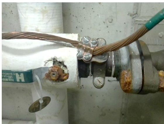
Plumbing: evidence of corrosion
