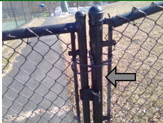
Fences / Enclosures: damaged gate latch
