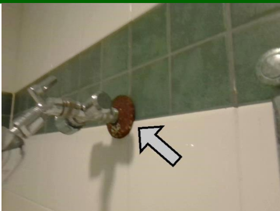
Womens Locker Room: example: corroded fixture
