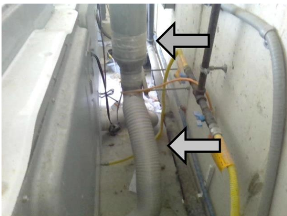
Laundry Facilities: dryer vent
