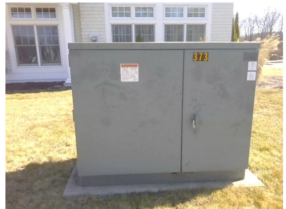
Electrical: transformer
