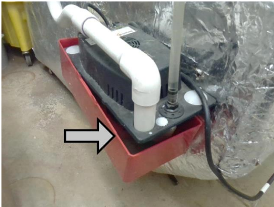
HVAC 3: damaged pump
