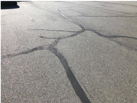
cracks have been sealed
