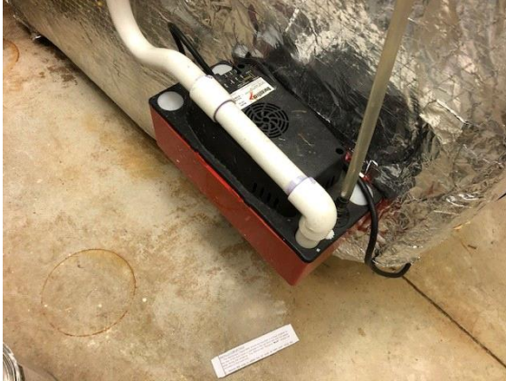
condensate pump replaced
