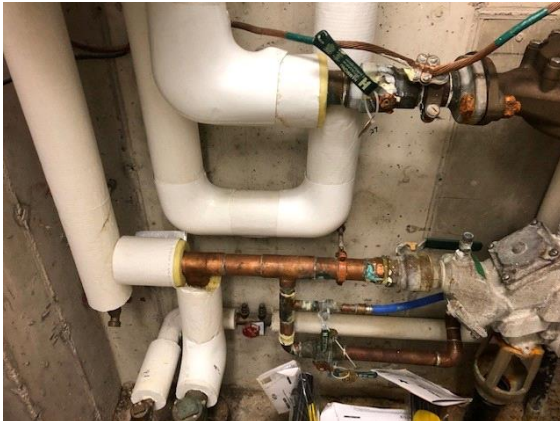
corrosion & leak repaired
