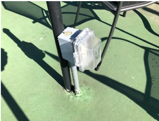
GFCI outlet & cover repaired
