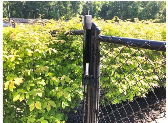
locking gate latch replaced
