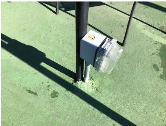
GFCI outlet & cover repaired
