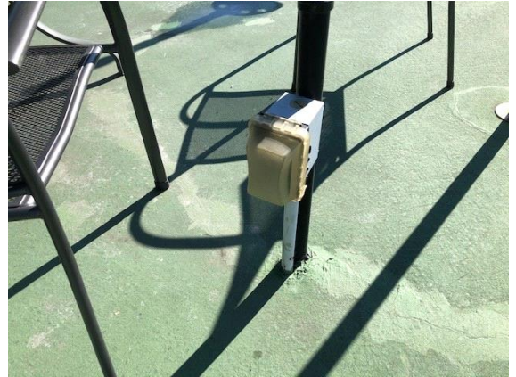
GFCI outlet & cover repaired
