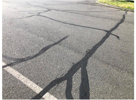
cracks have been sealed
