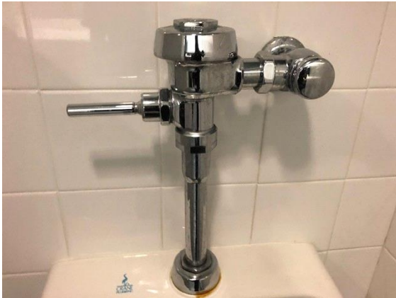
leaking flush valve repaired
