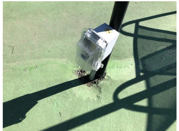
GFCI outlet & cover repaired
