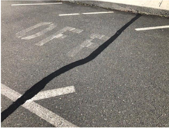
cracks have been sealed
