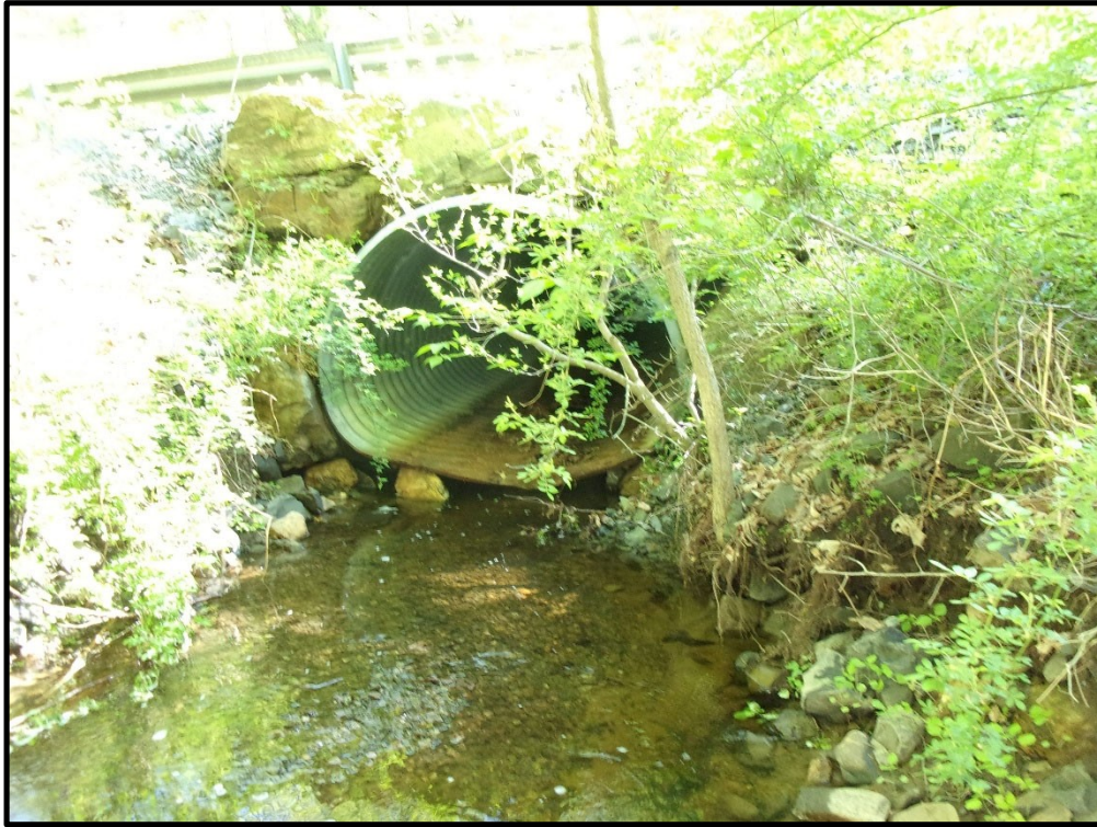
Downstream Bridge Elevation – Looking North. Note 14” perching.
