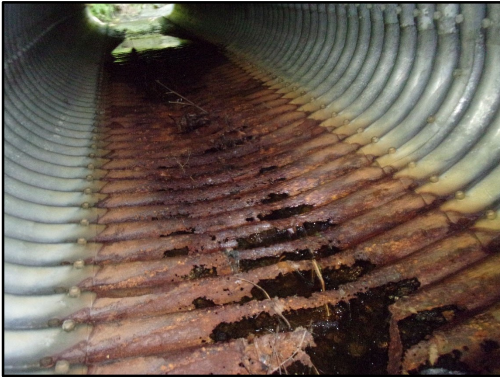
Pipe deterioration at outlet, up to 2' wide x full length with up to 100% section loss.
