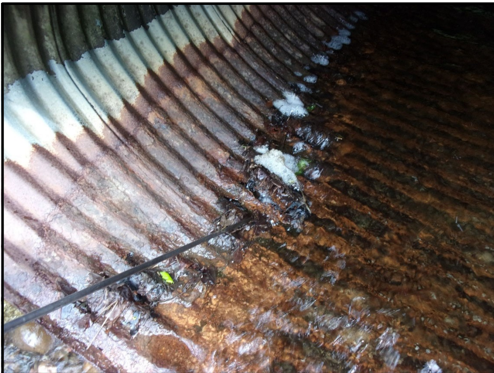
Deterioration at outlet. 100% section loss up to 6" long x 2" wide.
