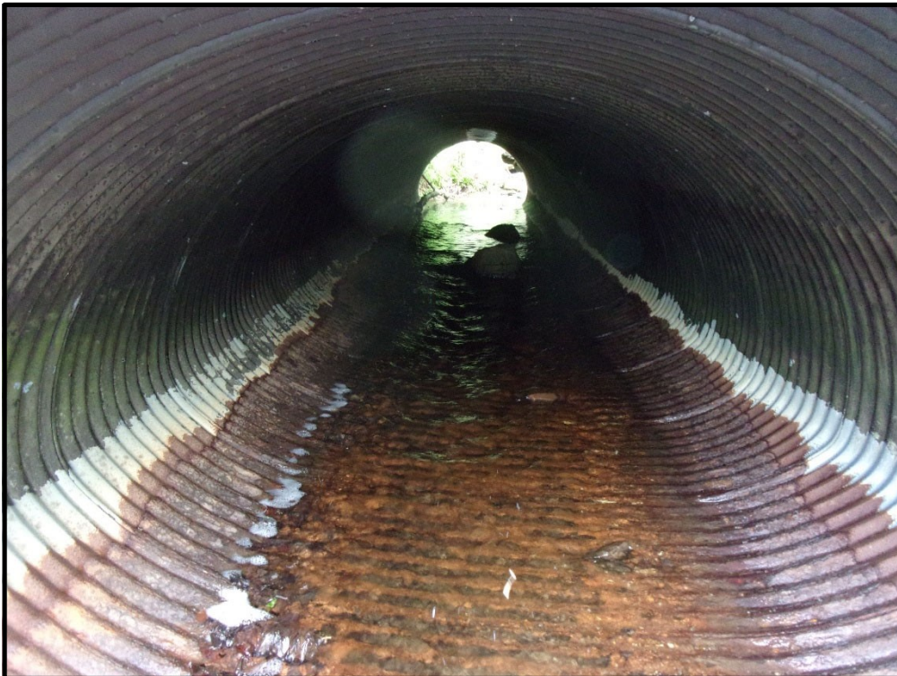
Pipe interior from outlet. Note heavy rust at invert.
