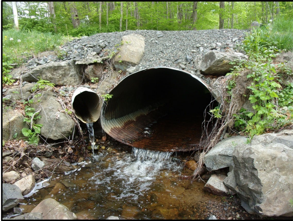
Downstream Bridge Elevation – Looking North. Note 6” perch at outlet.
