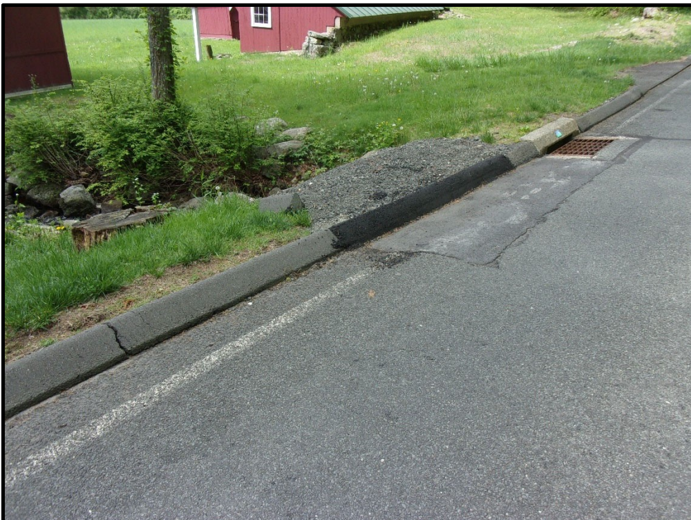
Roadway repair at downstream side. Note bituminous patch, bituminous curb and riprap.
