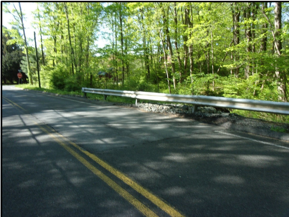
West side repair with riprap and bituminous roadway patch. Note no new curbing.
