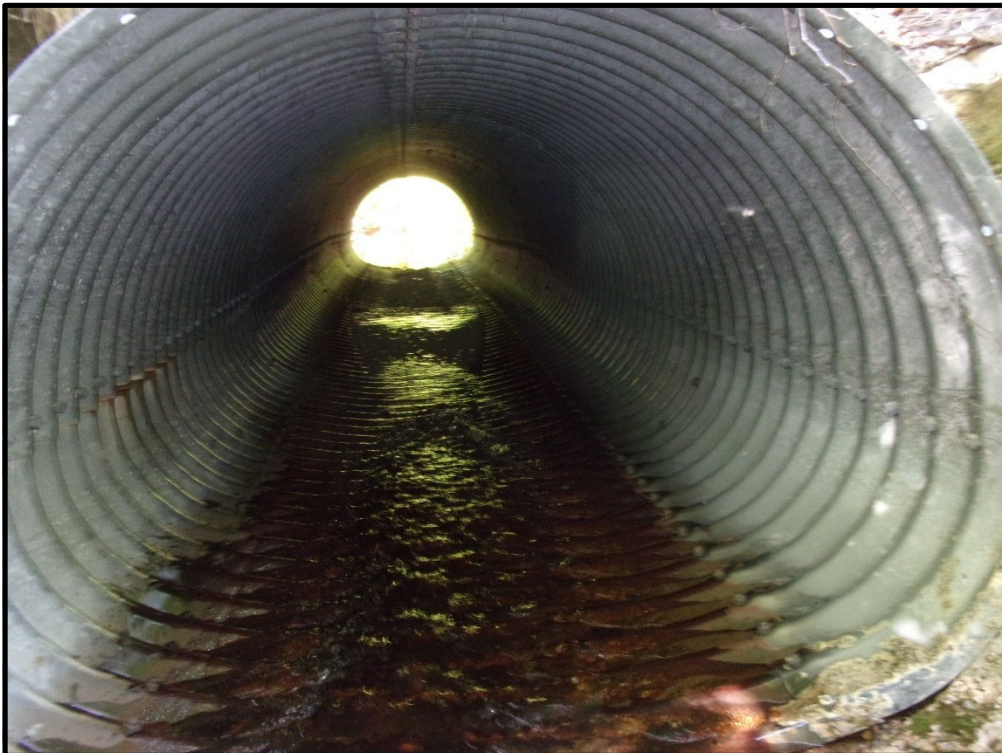
Pipe interior from inlet. Note deterioration along invert.
