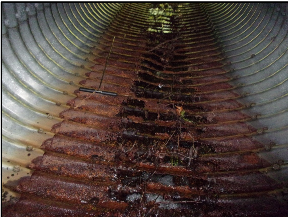
Pipe deterioration at outlet with up to 100% section loss. Note water flowing under pipe.
