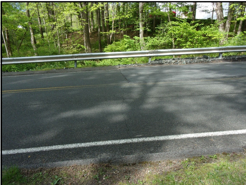
15' long hairline crack along east side of roadway opposite bituminous patch.
