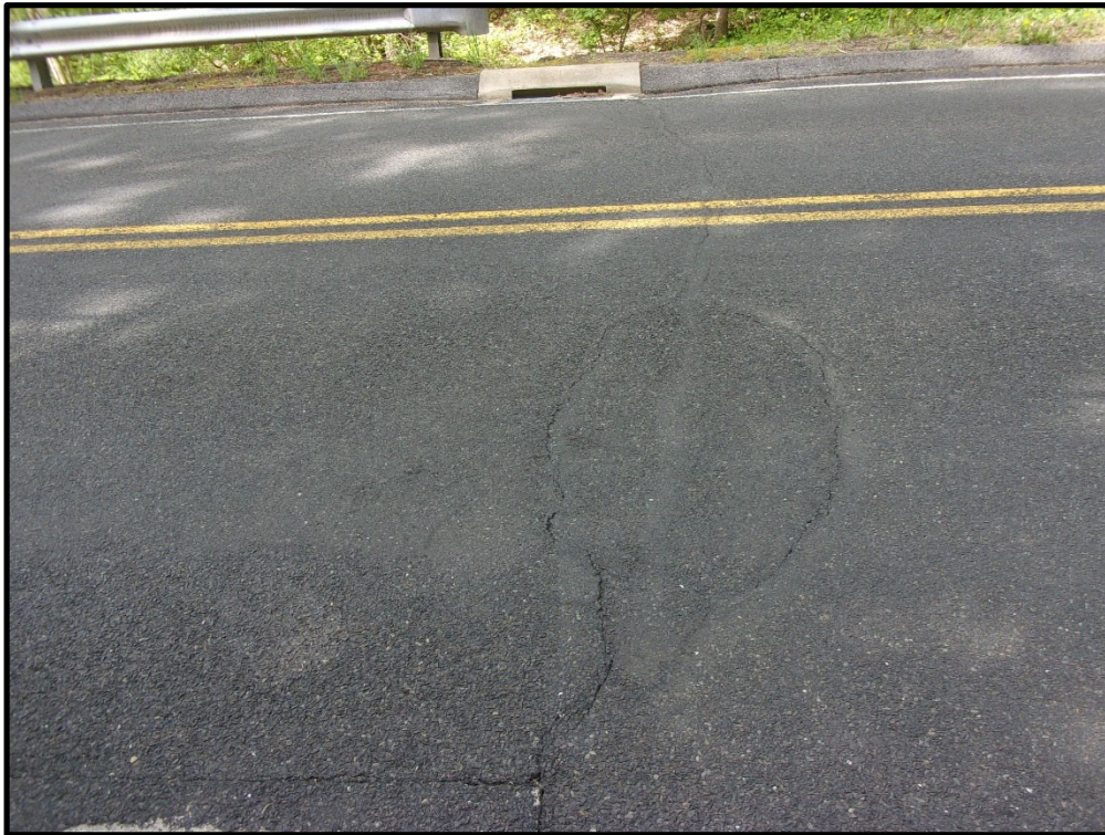
Bituminous patch and full-length hairline crack along catch basins, at north approach
